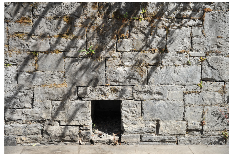
32 Three blocked up arches on Sheriff Street Lower 33 Infill stonework of arch
