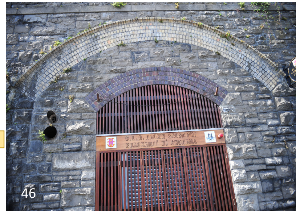
46. Entrance to vault on Seville Place
