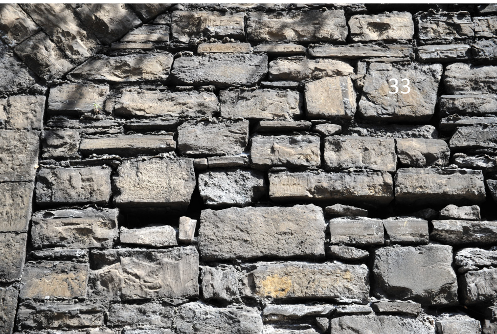
32 Three blocked up arches on Sheriff Street Lower 33 Infill stonework of arch
