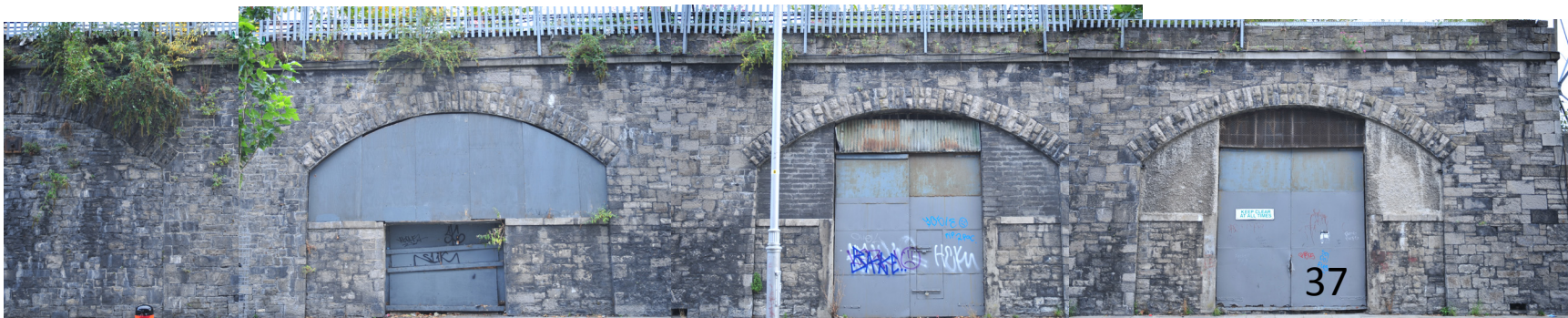
35 Workshop façade 36 Tie bars boundary wall at Oriel Street 37 Arches infilled either side doors Workshop building
