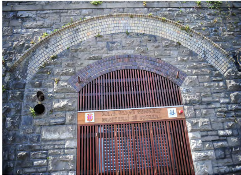
Vault at Seville Place
