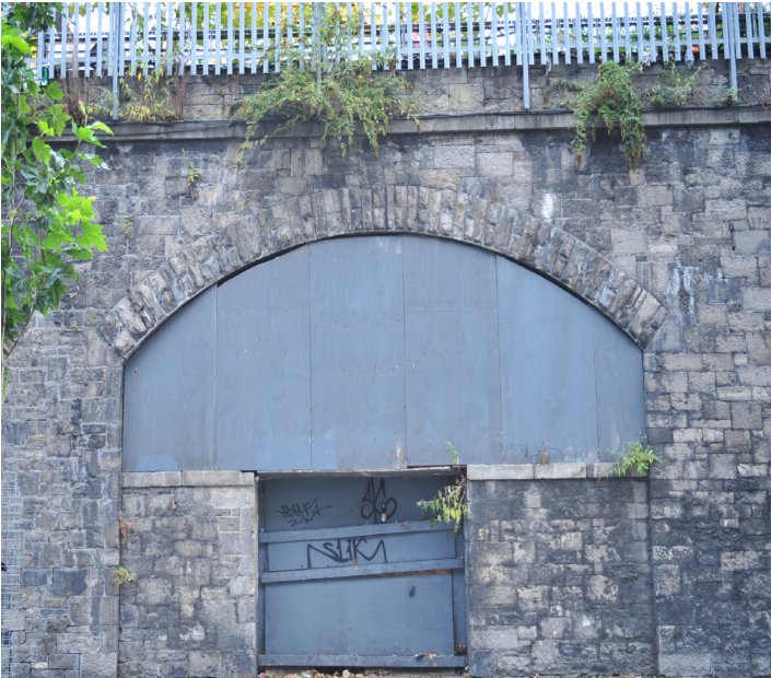
Protected structures clockwise from upper right 1. Infilled segmental arch of the flanking wall 2. Vault 9 Workshop 3. Oriel Street Upper boundary wall 4. Entrance to vault at Seville Place
