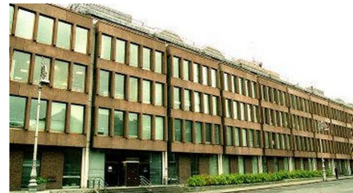
Planning permission for Stephenson's ESB headquarters was granted in full by Neil Blaney, Minister for Local Government, the day before the introduction of the new 1964 Planning Act. DOCOMOMO proposed its inclusion in the RPS.
