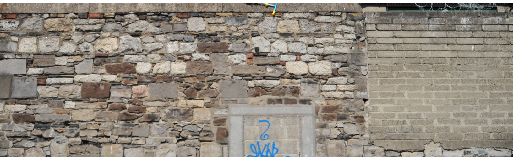
The wall has been rebuilt above the level of the infilled gateway head
